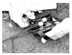
NOTE: All wires (supply and cold leads) must be inserted at the ends of the gel cap.
